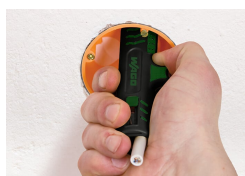
Stripping a cable sheath.
