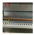
ERICO Connecting, Earthing and Neutral Busbars are used to connect several earthing conductors within a panel and can be used in a variety of different applications including switchgear and control equipment, electrical equipment, for wind and solar power generation and in data centers.
